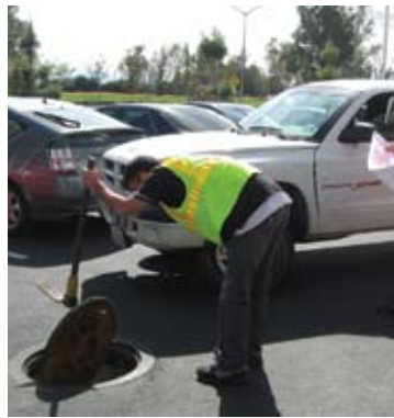
Left: Figure 3. Monitoring standing water for mosquitoes in a stormwater treatment system in Ontario, CA. Despite over a century of technological advancements, including air travel, space exploration, and the Internet, we still use pick-axes to remove manhole covers.
